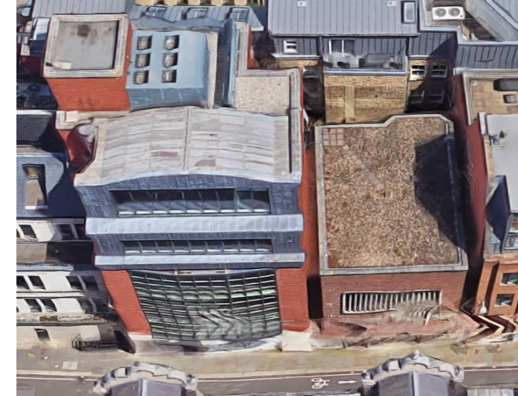
Figure 2-13 – Existing Site Showing 40-41 Furnival Street (Left) and 38-39 Furnival Street (Right)
