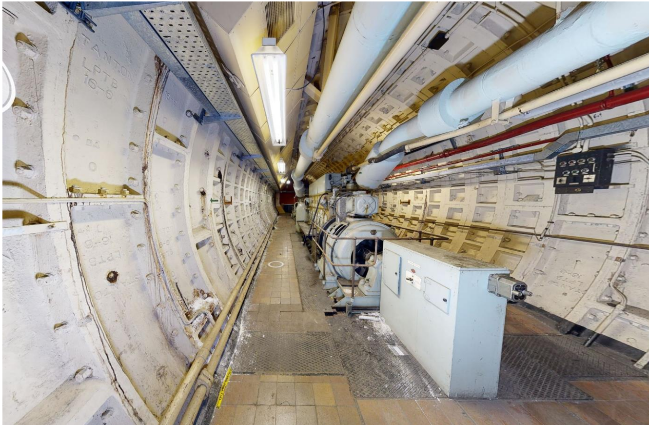
Figure 4-4 – South West Street – Existing Tunnel
