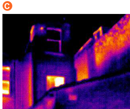
C The heat loss that is visible through the party wall indicates that 28 Willes Road is also experiencing severe heat loss. By building against this party wall, we will reduce heat losses from no. 28.
