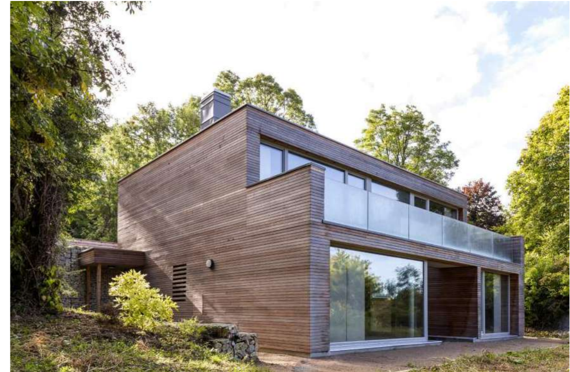
Figure 92. Lark Rise, UK's first Passive House Plus
