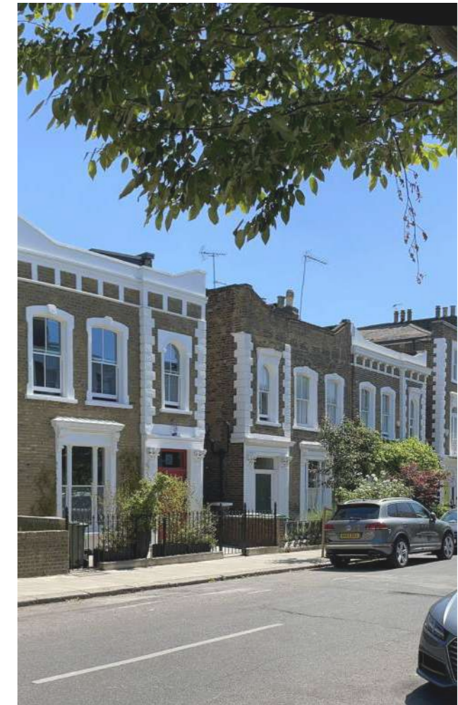
Figure 67. Panoramic street view of existing house, showing the plaster detailing that has been lost along the top of the front elevation
