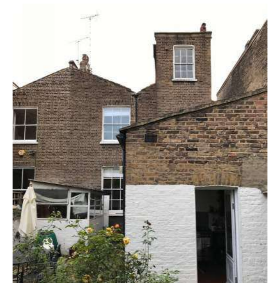
Figure 15. View of back wall from garden
