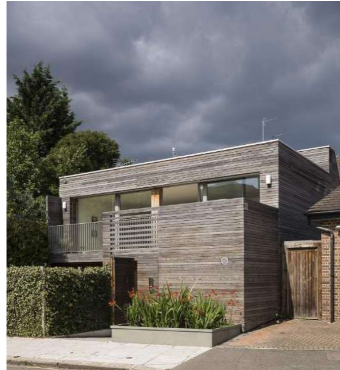
Figure 91. Camden Passivhaus, England's first Passive House
