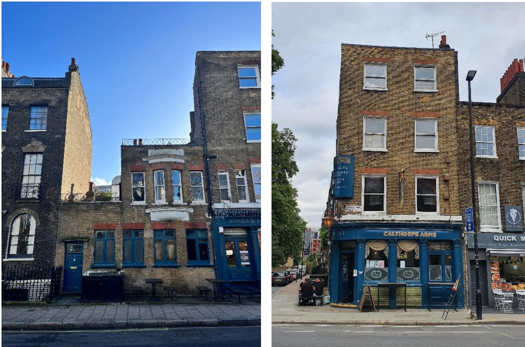
Fig 15 and 16: View of site from Wren Street and Grays Inn Road, respectively.
