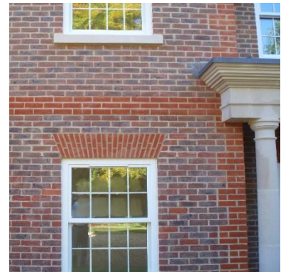
Fig 27: Flat gauged soldier course/ arch.
