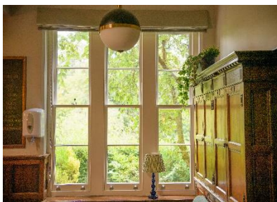
Fig 31: painted timber 1 over 1 sash windows.
