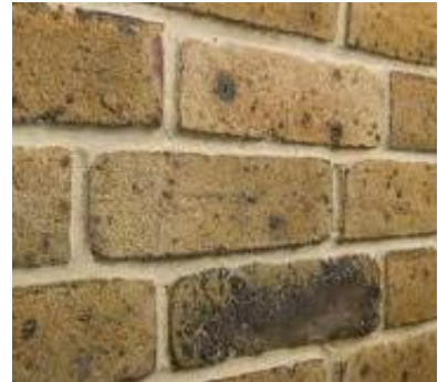
Fig 30: London stock brickwork to match existing.
