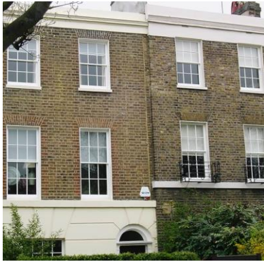
Fig 25: Painted timber 6 over 6 sash windows.
