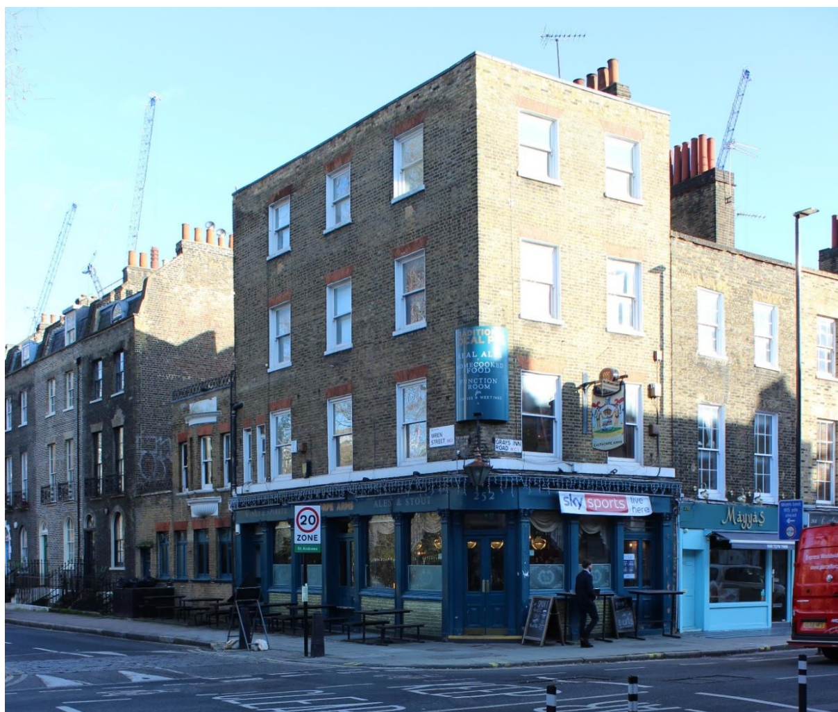
Fig. 8: View from the west with Wren Street to the left and Gray's Inn Road in the foreground (18 January 2023).
