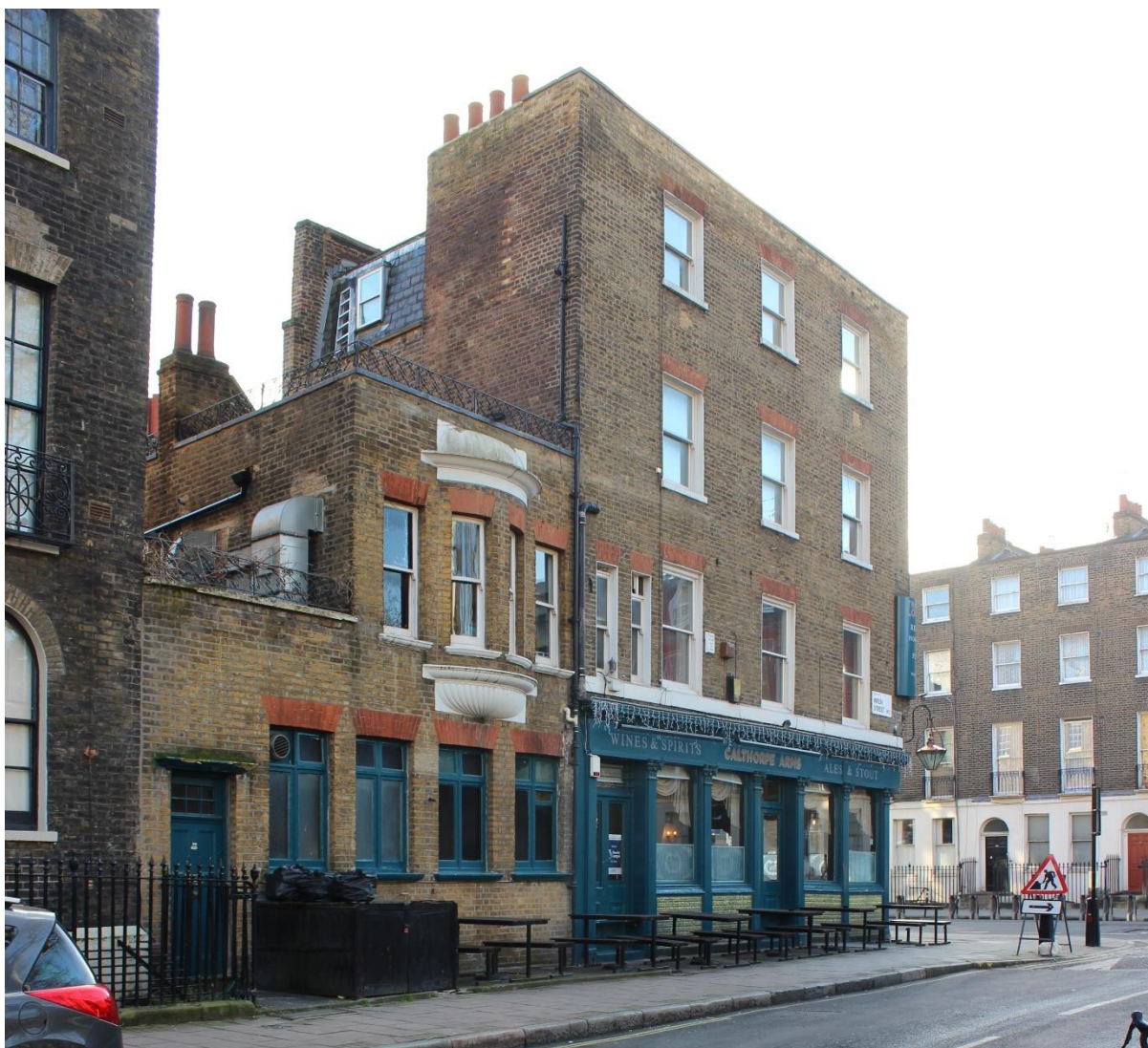
Fig. 9: View from Wren Street (18 January 2023). Note the flues on the side of the extension.
