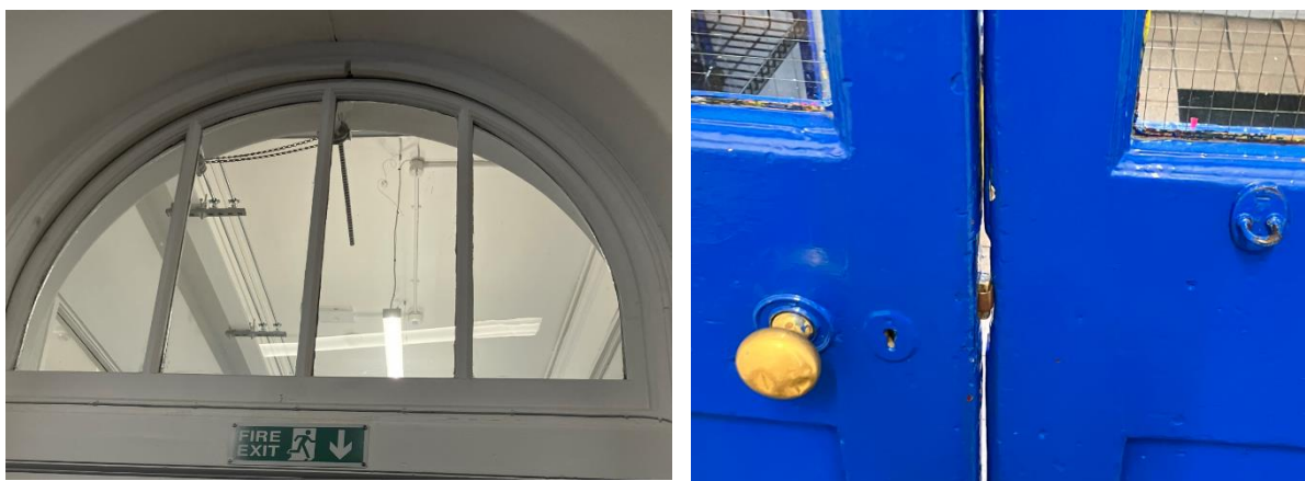
Figures 2 and 3: non fire rated glazing to be replaced & Damage to door leaf allowing passage of flames/smoke
