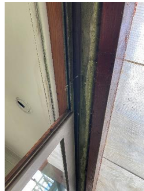
E.2 – Single glazing to rear windows.
