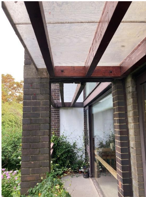
E.5 – Existing balcony and timber shelter / brise solei
