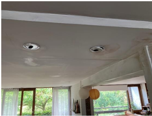
E.1 – Dropped ceiling to allow recessed lights.
