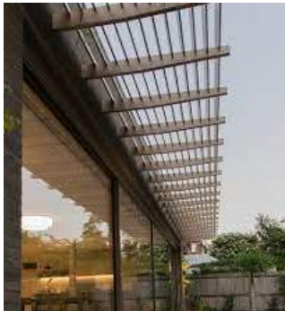
External brise solai. Similar shading can be achieved with balconies.
