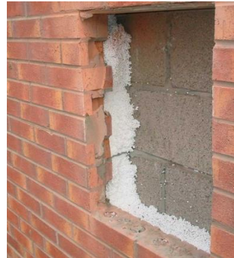
Example of EPS beads than have been blown into a cavity wall.
