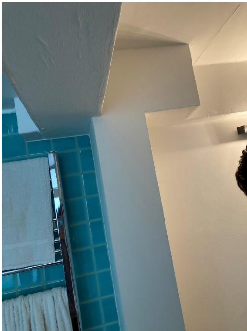
E.7 – Lower ground floor – boxing out to route drainage.
