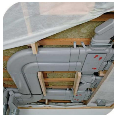
Zhender flat ductwork system.
