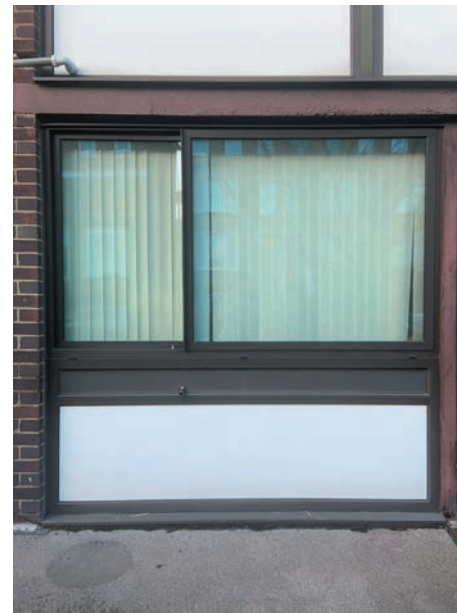
View of the Aluminium glazing at front
