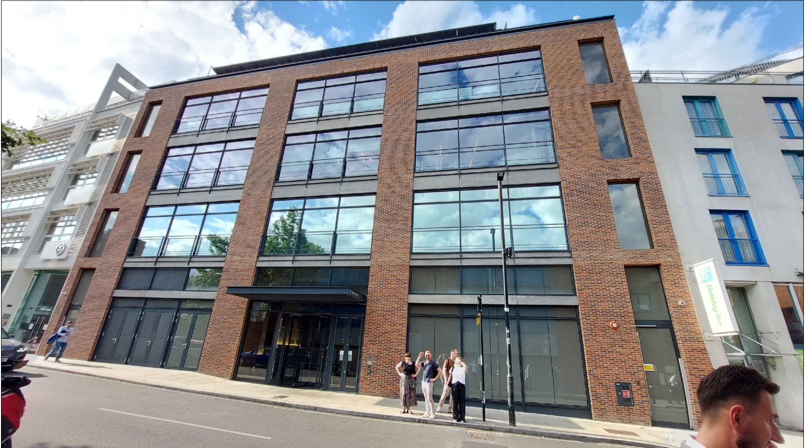
EXISTING VIEW SOUTH ELEVATION OF 32 JAMESTOWN WHARF
