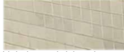
Light brown brickwork
