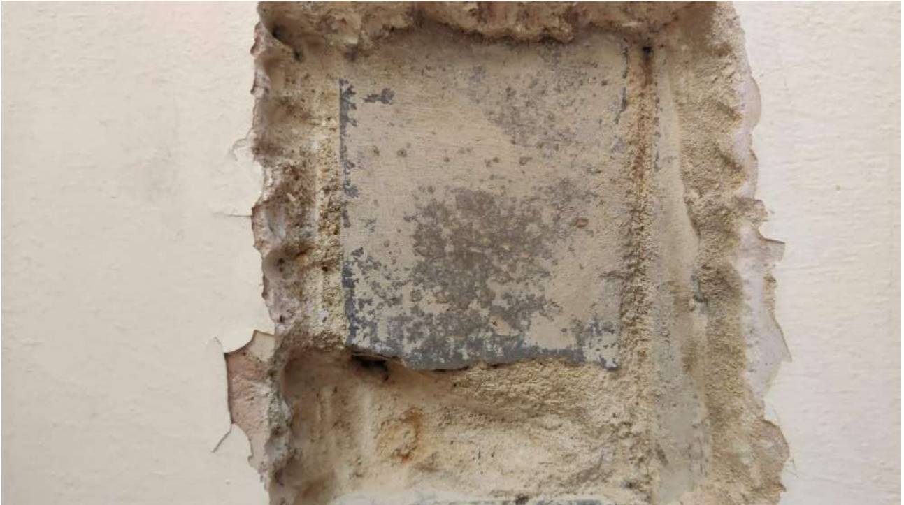
Opening up works showing area of modern brick pier.
