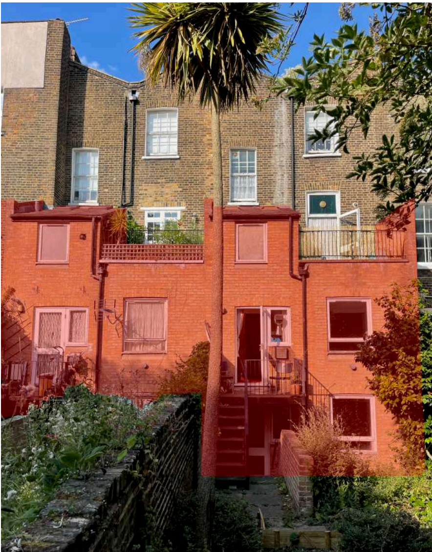
Modern extension on rear elevation
