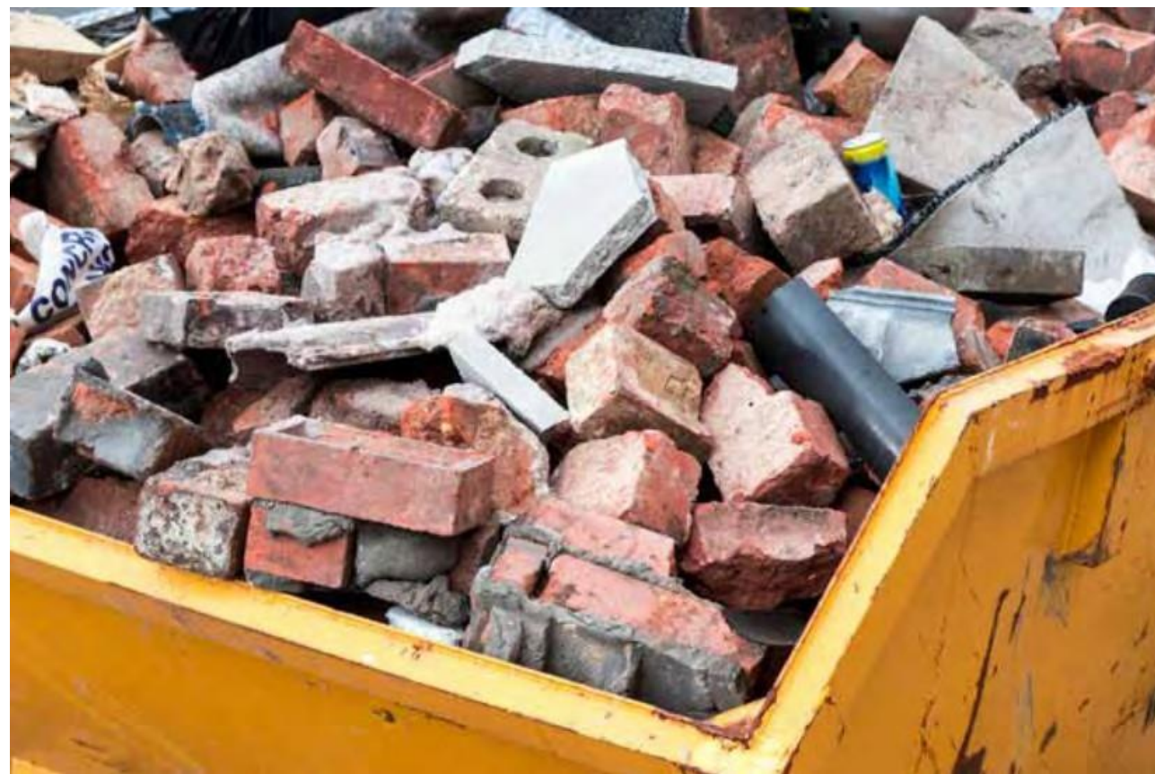
Typical Demolition Waste in a Skip - Mixing of Such Products Diminishes Their Recovered Value
