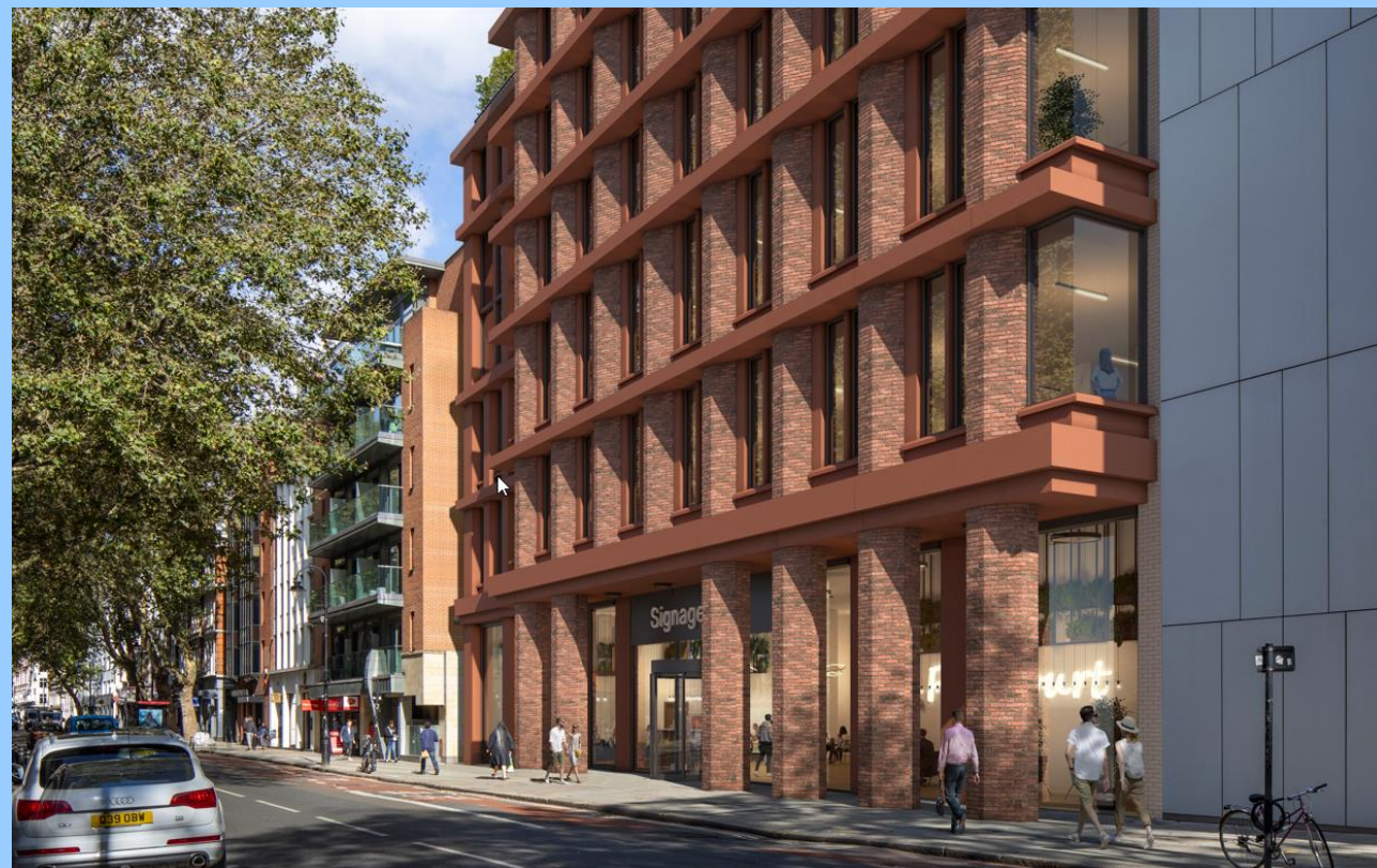
Architect's CGI Image of the Fox Court Redevelopment from Gray's Inn Road
