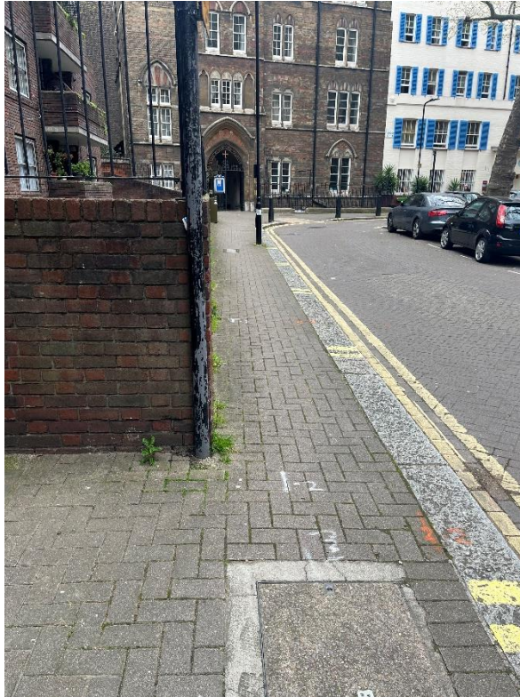
Photo 7: Brooke Street Adjacent to Footway
