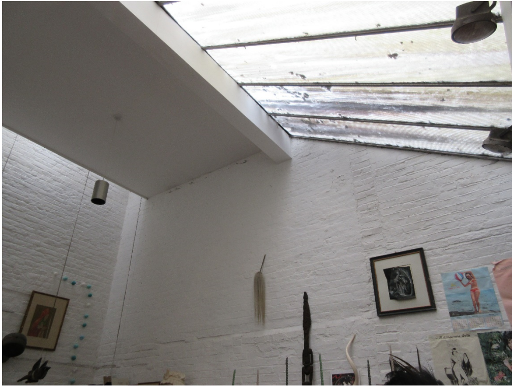
Inside rear extension studio (photograph dated 2019)
