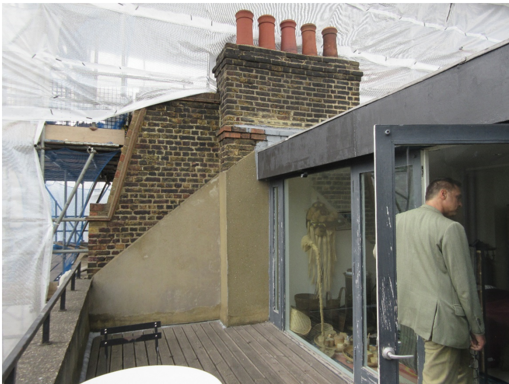
Existing roof (photograph dated 2019)
