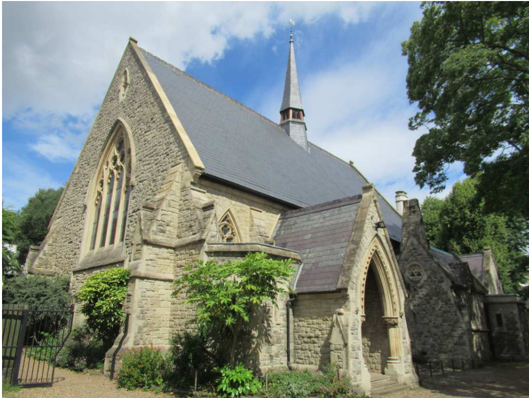
Image 2 – South Elevation, porch
