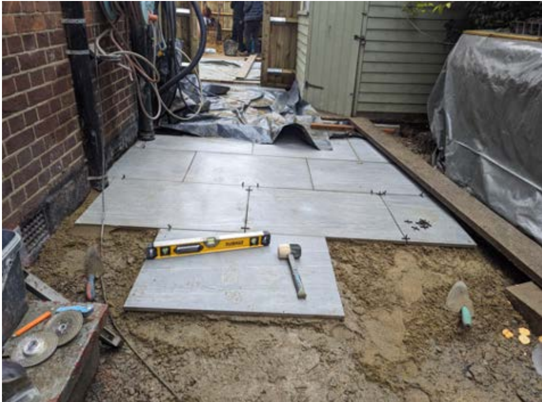
Image 3: Partially Installed Hardstanding Source: Viable Placemaking Site Visit
