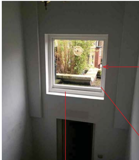
Modern reduced height window due to rear closet wing below
