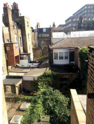
View from the rear of 41 Doughty street
