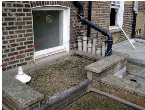
Non original stair window blocked by later addition closet wing
