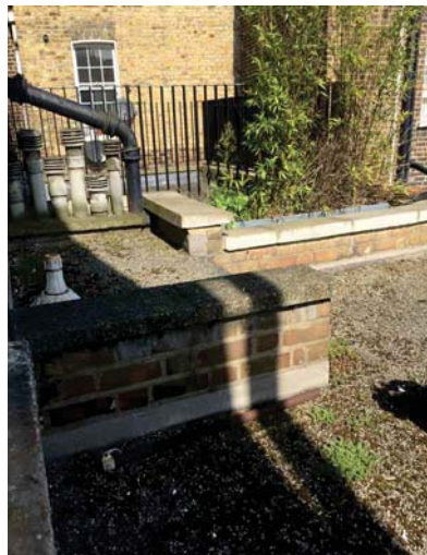
View from the rear of 41 Doughty street
