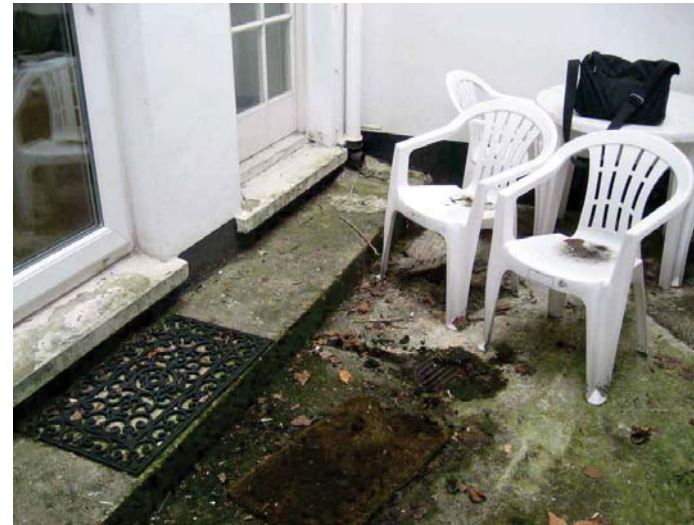
Rear external space at LGF level accessed via 1970s rear extension
