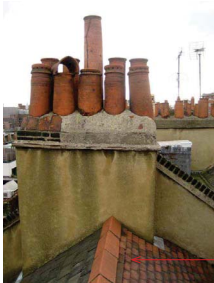
Slate to street slopes badly weathered
