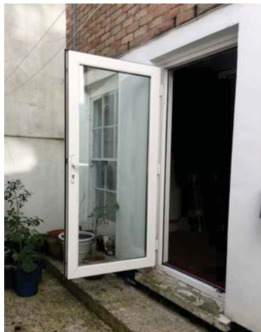
LGF modern interventions
