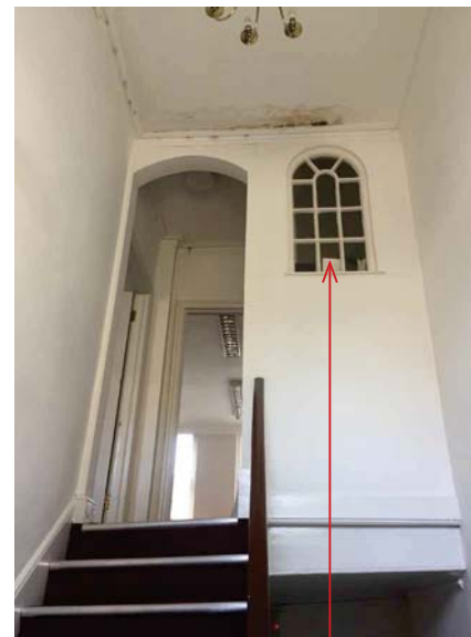
Partition wall at head of Second Floor staircase with poorly detailed glazed element
