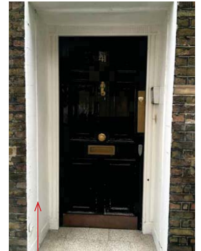
Original position of entrance door
