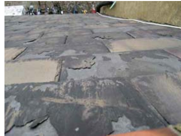
Slate to outer valley with red clay tile to internal slopes
