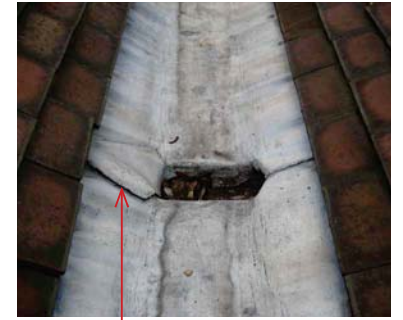
Leadwork welding to gutter outlet lifting
