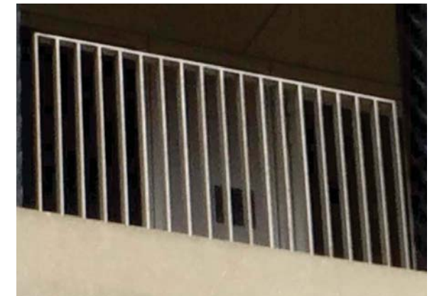
Balustrade: Narrow mild steel sections as per Chipperfield balustrade example
