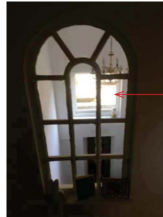
Modern reduced height window due to rear closet wing below
