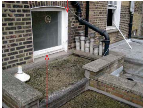
Window height reduced due to closet wing below
