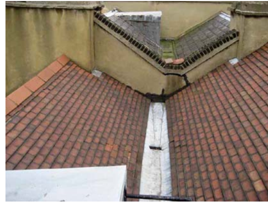
Leadwork welding to gutter outlet lifting
