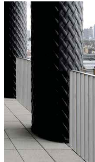
Balustrade: Narrow mild steel sections as per Chipperfield balustrade example
