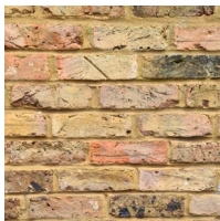
Reclaimed London Stock brickwork with pointing to match existing
