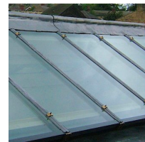
Standard patent glazing to match the existing glazing above the existing lean- to structure
