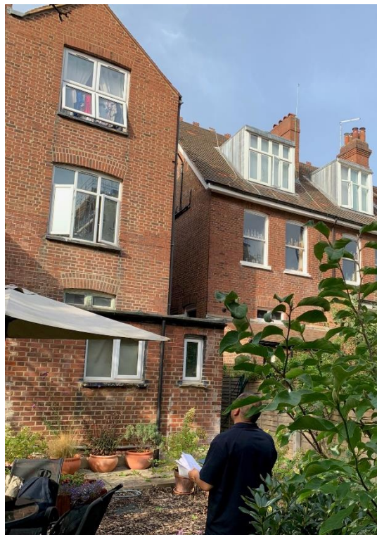
Photograph 4: Looking towards No.8
