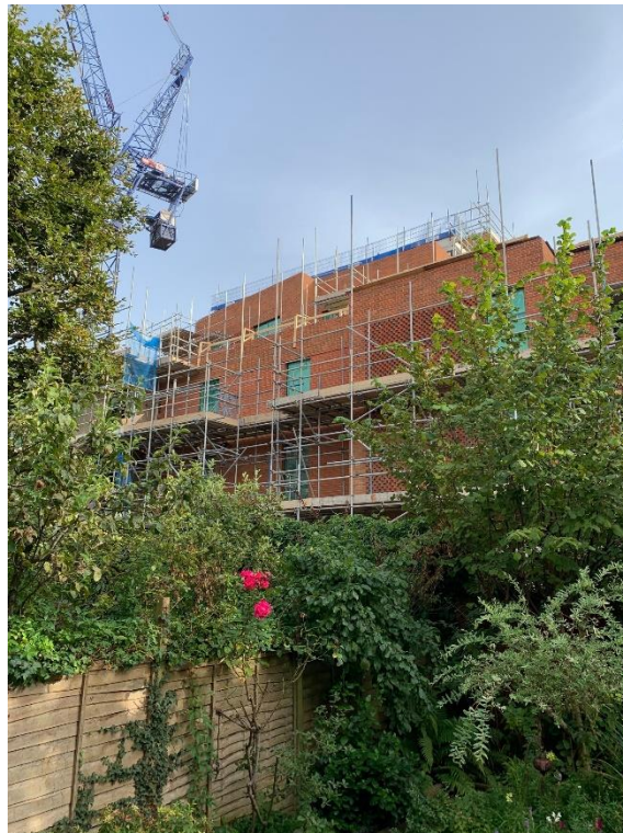
Photograph 5: Development to the rear of the site
