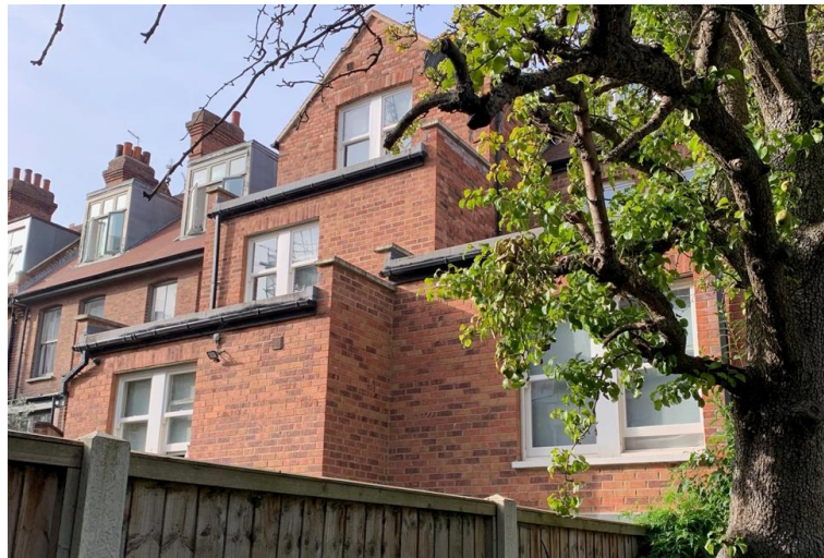
Photograph 3: Rear of No.12
