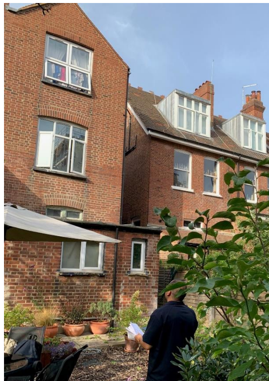
Photograph 4: Looking towards No.8
