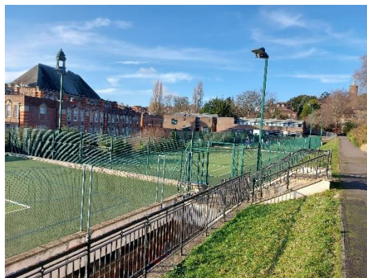
Plate 4.11: Tennis Court Roof
