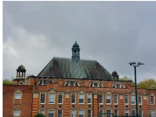
Plate 4.3: Building B2 Roof
