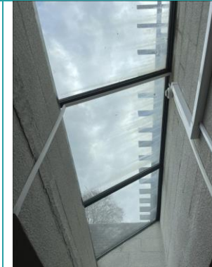
Image 17 GS Wing - Metal Skylight Frame
