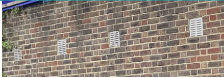
Image 14 Fives Courts - Metal Vent Grills
