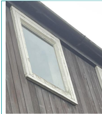
Image 49 Fives Courts - Single Glazed Window
