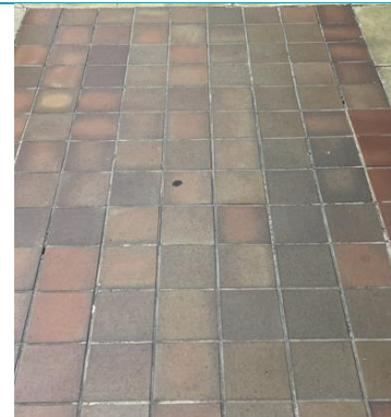
Image 46 GS Wing - Quarry Tiles
