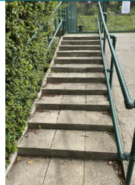
Image 28 External Areas - Metal Key Clamp Railing
