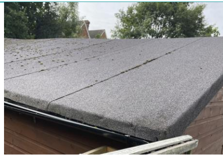
Image 66 Maintenance Shed - Mineral Roof Felt
