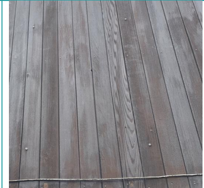
Image 32 Fives Courts - Timber Panelling
