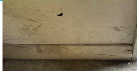
Image 30 Fives Courts - Timber Skirting
