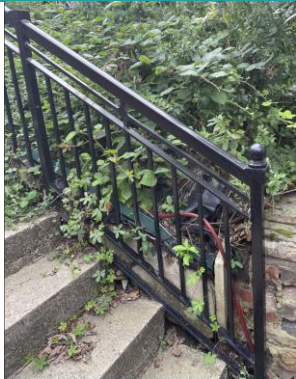
Image 26 External Areas - Metal Railings
