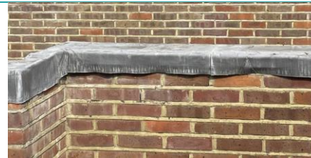
Image 20 GS Wing - Leadwork
