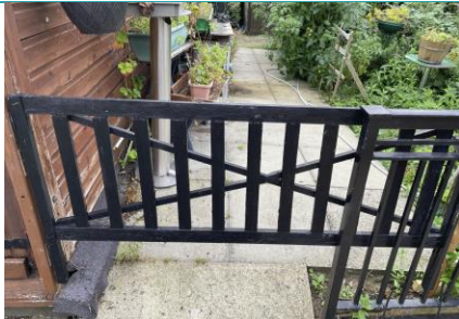
Image 33 Maintenance Shed - Timber Gate
