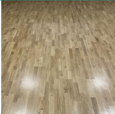
Image 29 Fives Courts - Timber Floorboard
