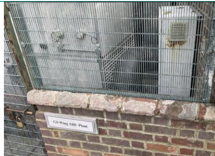
Image 19 GS Wing - Steel Mesh Fencing
