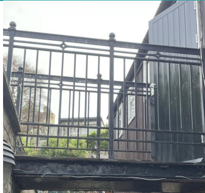
Image 27 External Areas - Steel Bridge Walkway
