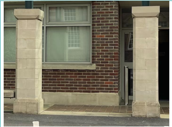
Image 63 GS Wing - Stone Cladding
