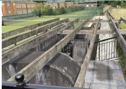
Image 42 GS Wing - Timber Roof Plant Room
