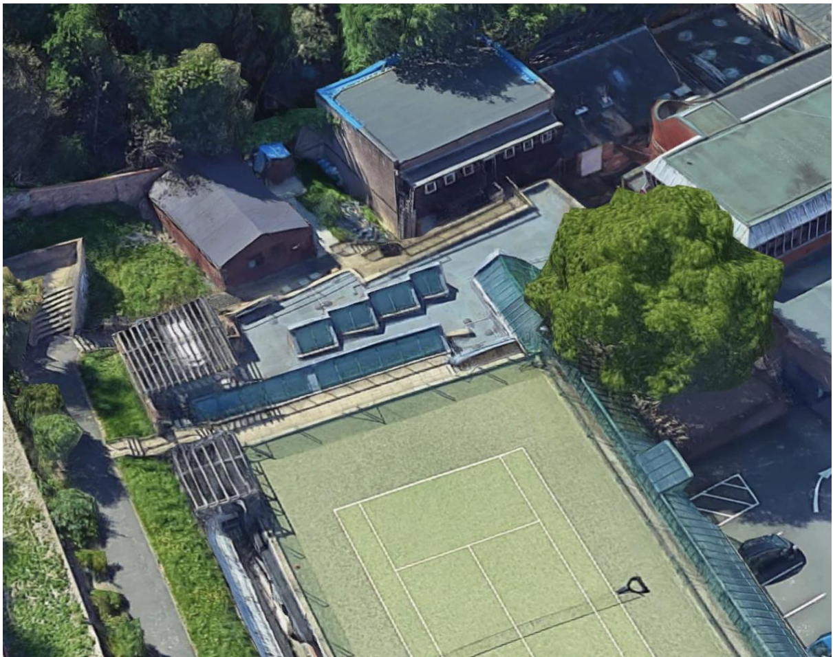
Aerial GoogleMaps bird's eye view from north-east of 3 buildings
