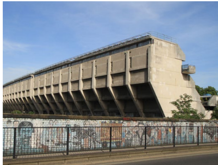
Block A north facade from Abbey road
