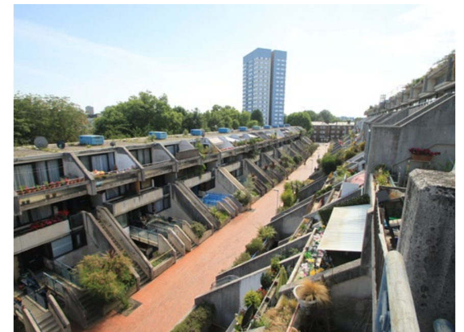
View South-Wet to block B from Block A Staircase
