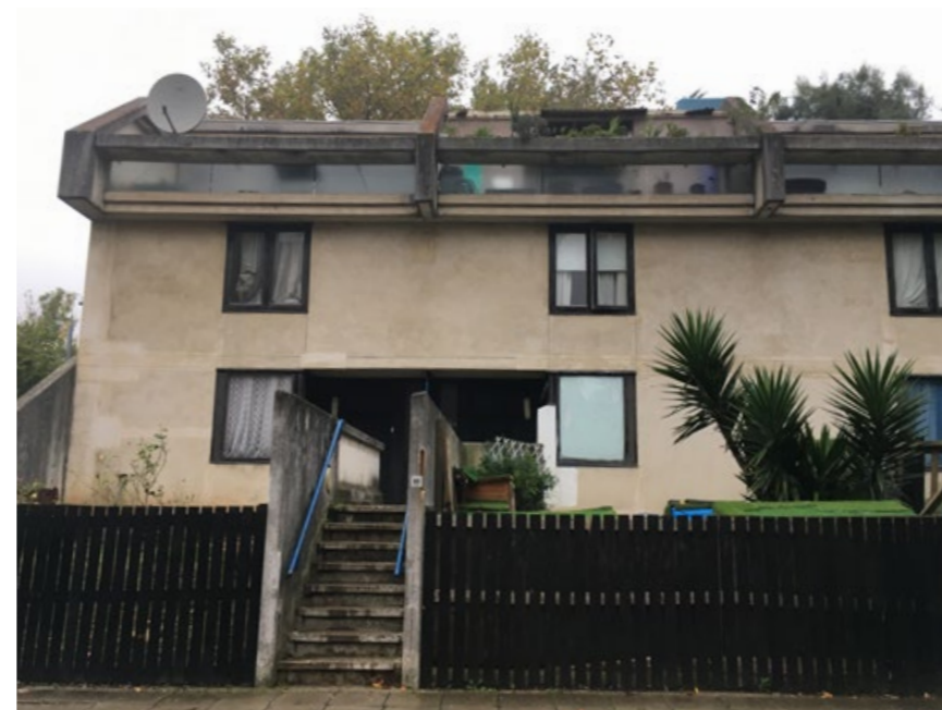
Block C from Boundary road (South elevation)
