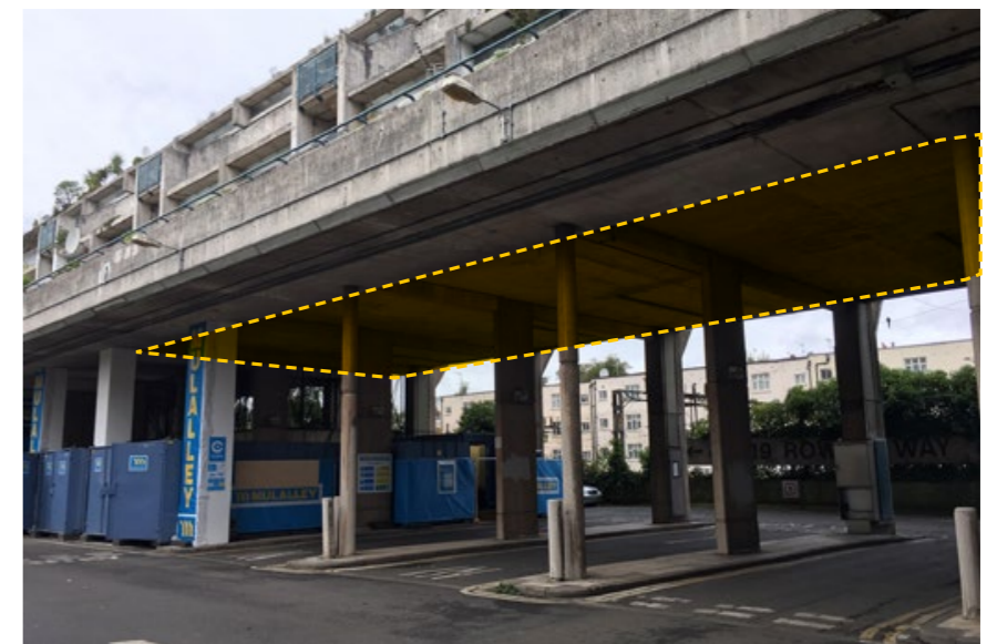
Figure 4.3 - Exposed floors at the eastern end of block A
