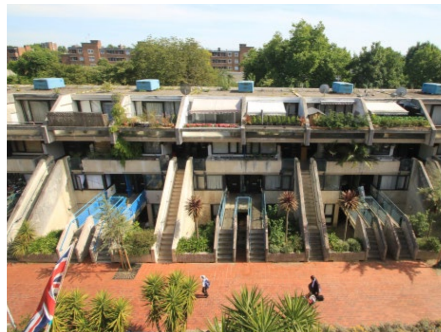
Block B North elevation, Rowley way, seen from Block A
