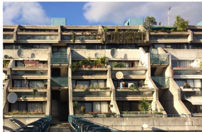
Figure 3.1 - Block A - south stepped facade
