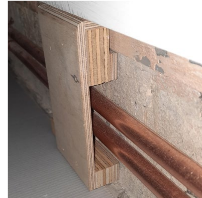
Proposed skirting section in pilot flat
