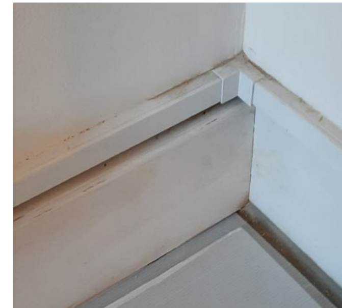
Proposed finished skirting board in pilot flat
