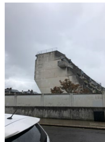
Figure 3.3 - The western end wall of block A illustrating heat loss from the dwellings and significant thermal bridges at the floor and wall junctions.
