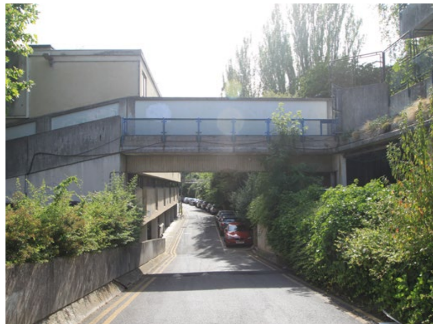
Link bridge between TRA Hall and block C
