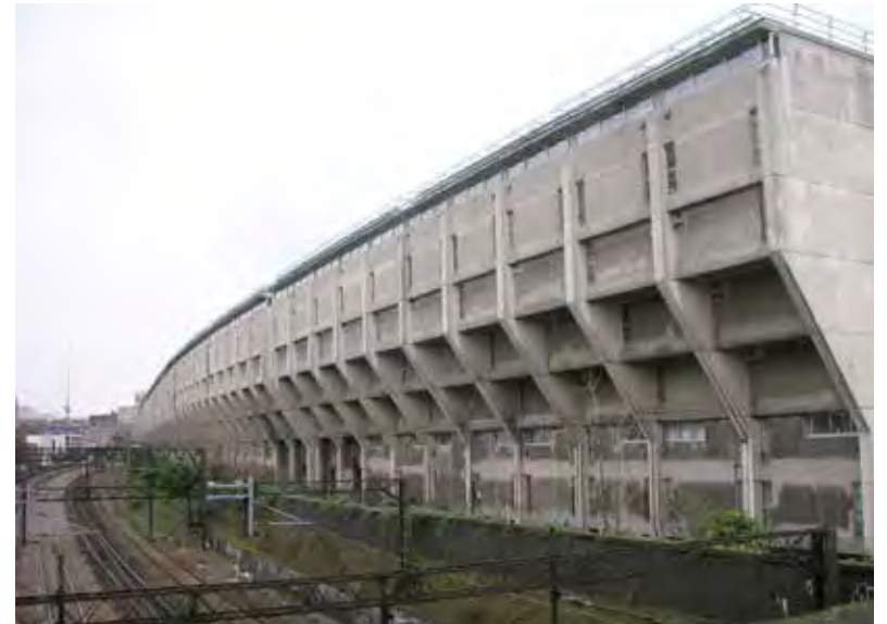
Figure 2.9 - Rear of Block A
