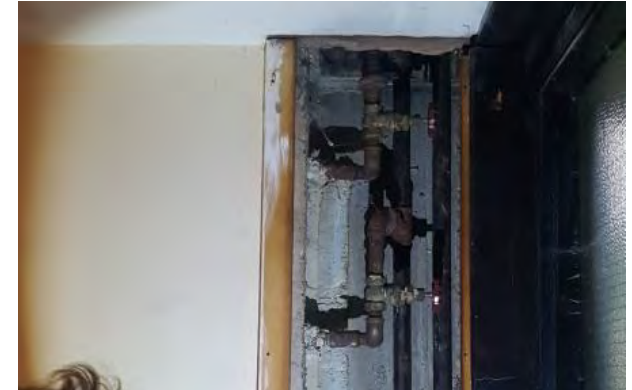
Figure 5.2 - Alexandra Road heating network inspection
