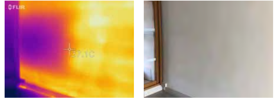
Figure 11: Internal image of the same void A1 unit, showing the coil heated party wall - facing towards the railway line. It is possible to see the route of the tail pipes at the top and bottom of the wall from the heated coil.
