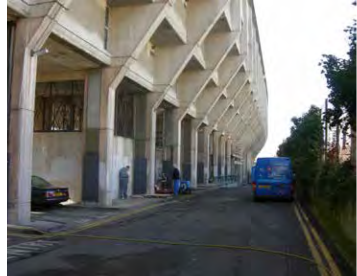
Figure 7.4 - Block A - rear facade
