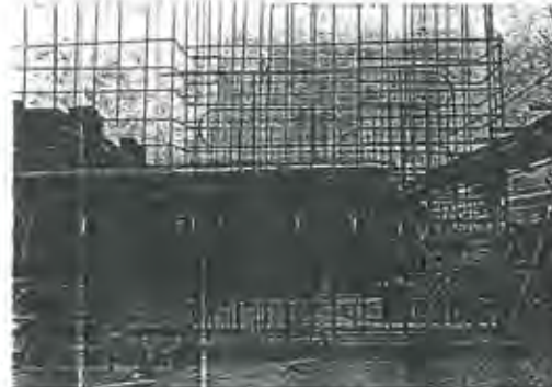
Fig 3 - Steel pipe coils in position before casting the concrete
