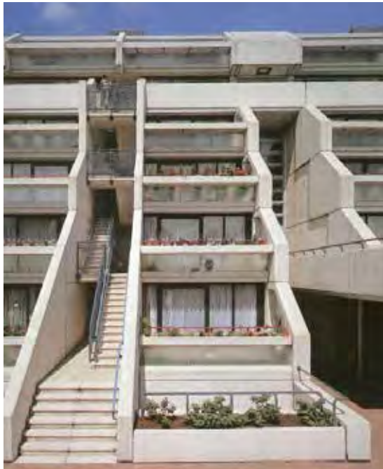
Figure 2.2 - Block A South elevation
