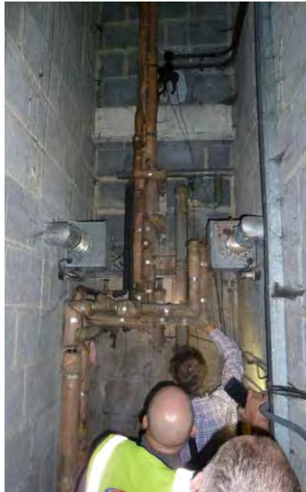
Figure 5.0 - Alexandra Road heating network inspection
