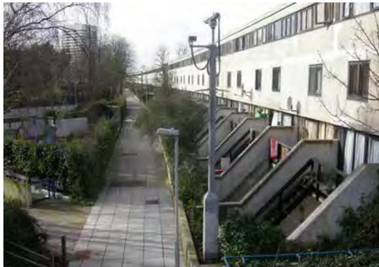
Figure 2.11 - Rear of Block B
