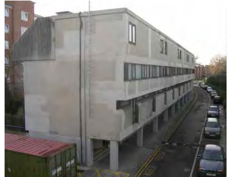
Figure 2.12 - Block C facing Ainsworth Way
