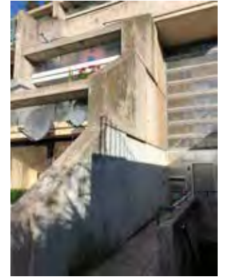
Figure 7.2 - Eastern end wall of block A illustrating heat loss from the heating coils in the dwellings.
