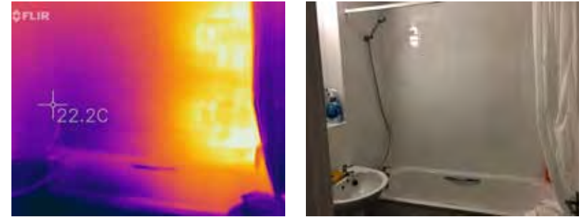
Figure 16: Image of the bathroom wall in same A3 void unit on the lower floor showing the heating coils and likely zone for the tails.
