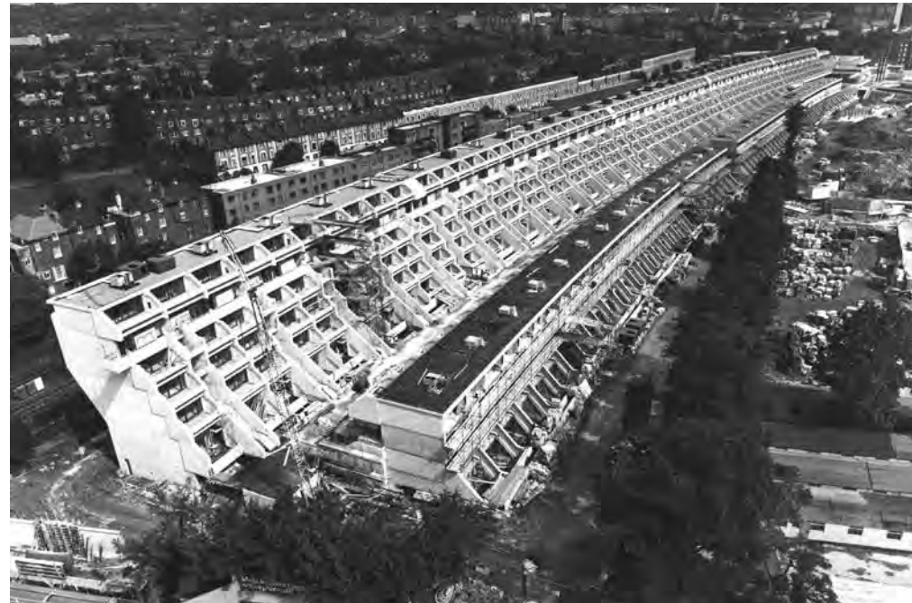
Figure 2.3 - Aerial view of Rowley Way and Langtry walk under construction
