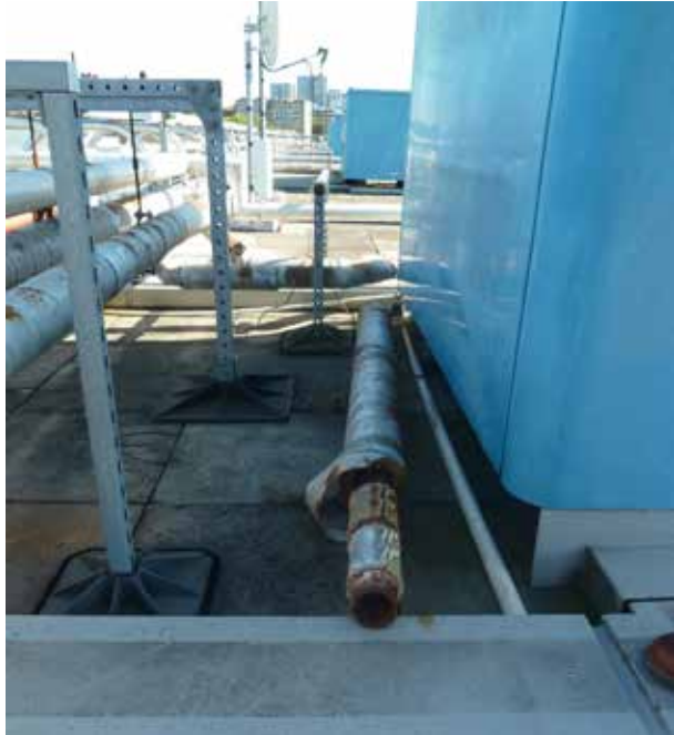
Figure 4.0 - Condition of heating pipes located on the roof of Block A
