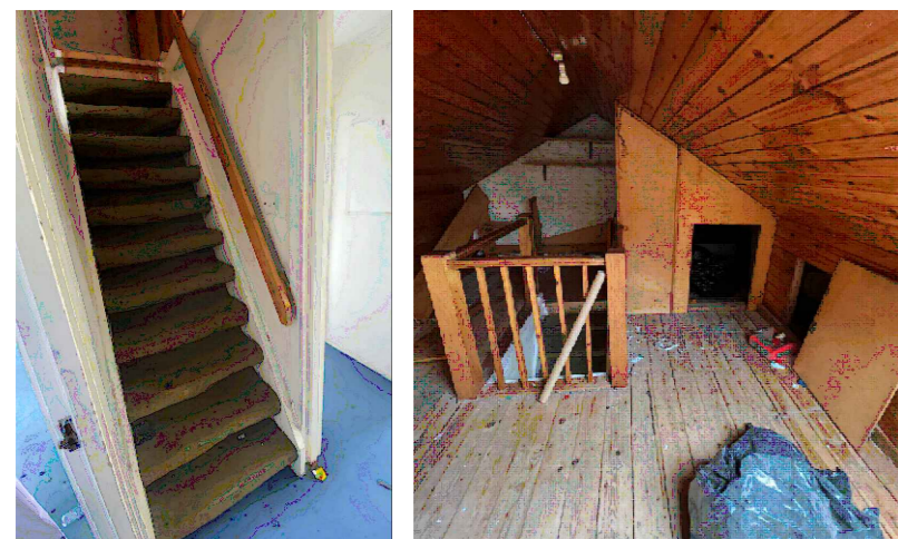
EXISTING 3rd FLOOR AND LOFT PHOTOS, APRIL 2023
