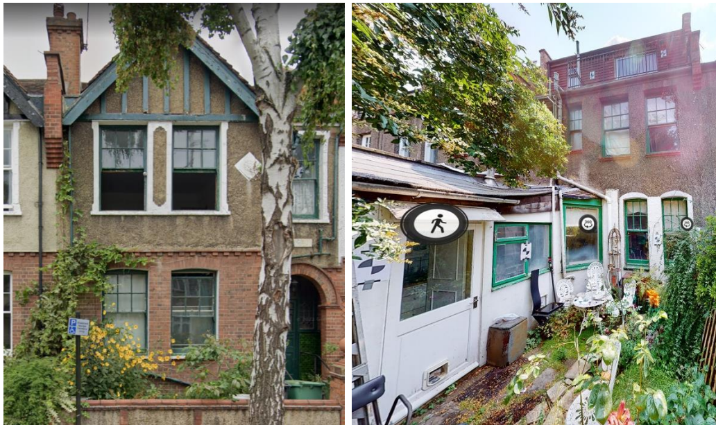
Figure 07. Existing front and rear façades of 32 Glenhurst Avenue
