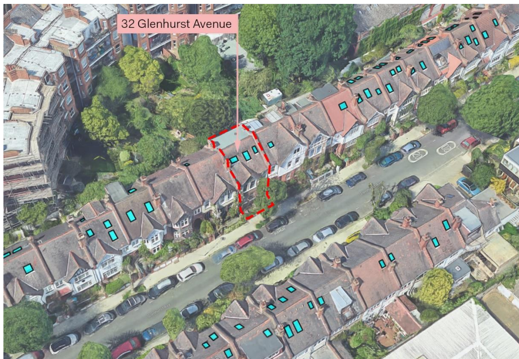
Figure 06. Existing rooflights on the neighbouring properties
