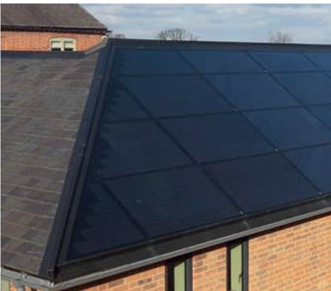
PV solar roof panels
