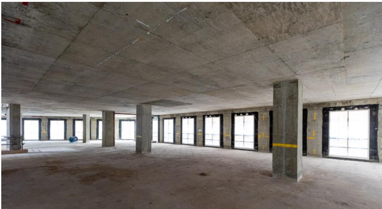
Figure 12 - Soft stripped completed on recent ECL scheme
