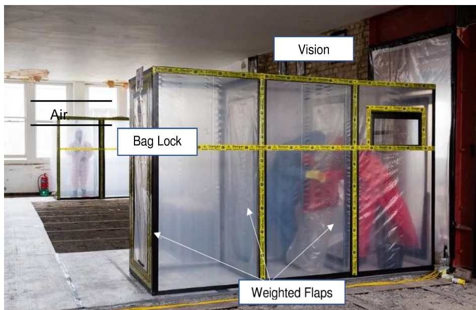
Figure 10 - Air lock construction for fully controlled zone
