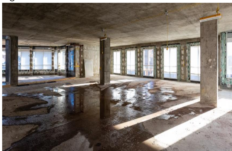
Figure 13- Dampening down during soft strip works
