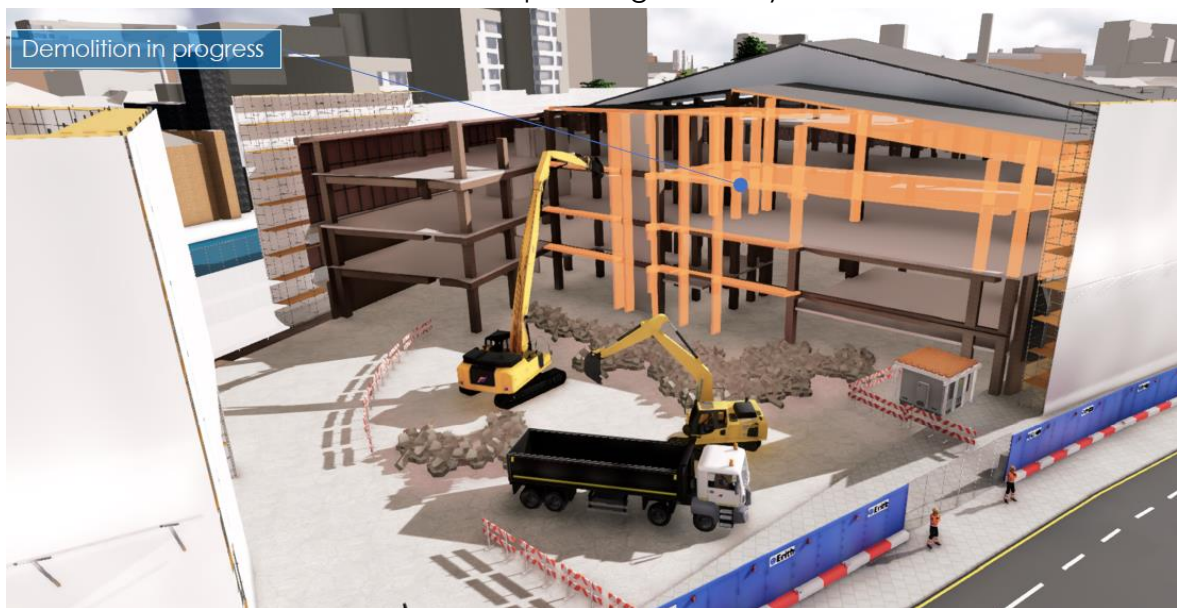
Figure ? – Block C demolition progressing
