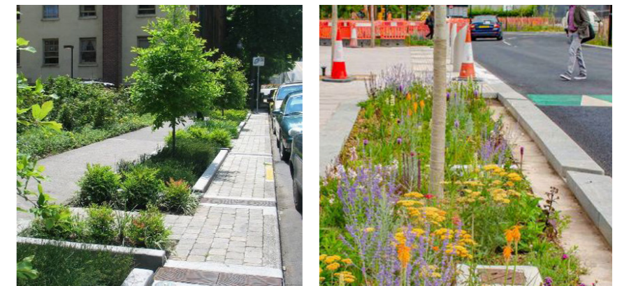
Examples of Rain Gardens that maintain a 0.6m setback from kerb edge.
