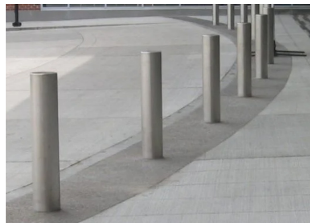
O1 When there is the absence of a mound, the security line is supported by bollards
