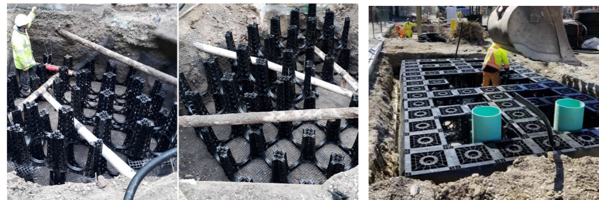
Examples of Greenblue Urban work with planting over existing utilities.
