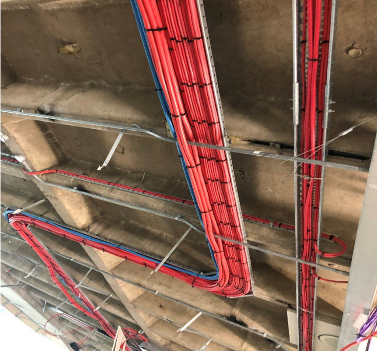
Level 24 multiple cables running through the floor to old VA rack now being used as a joint box
