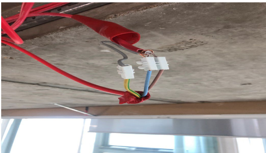
Pyro joint causing short circuit due to earth link touching both pairs
