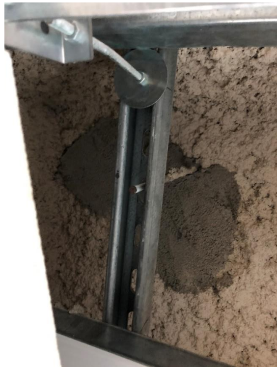
Figure 7: Small patch repair
