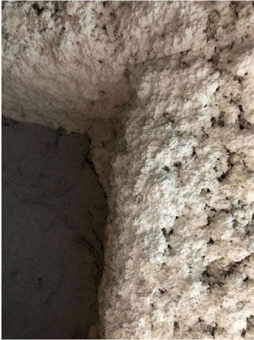
Figure 8: Large patch repair
