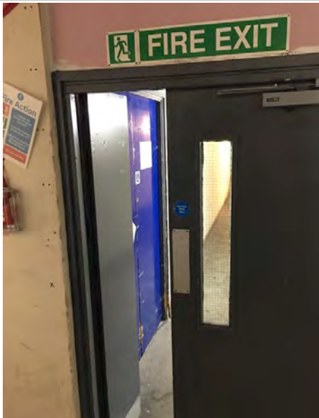
A self closer should be added to half leaf of door.
