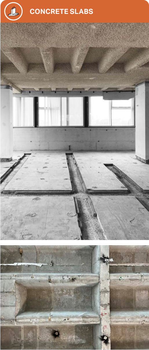
Figure 4.3 Ribbed concrete slabs at Euston Tower
