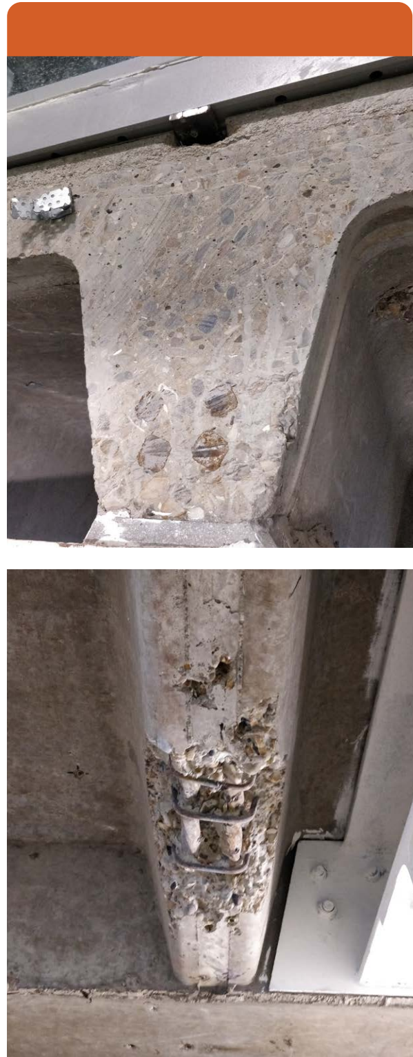
Figure 3.8 Images of existing ribbed slabs
