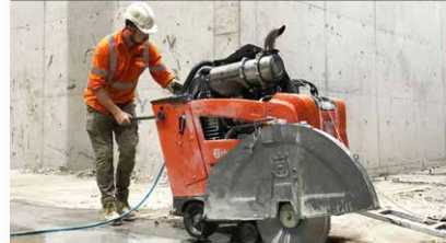
Cutting out and reusing in-situ concrete ribbed slabs (reference image)
