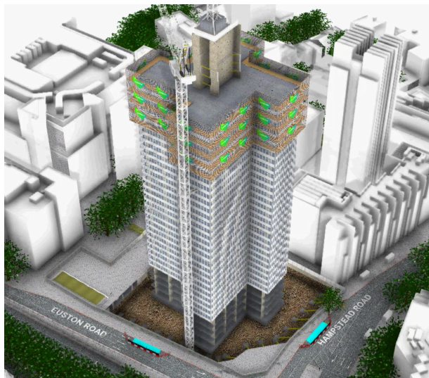
a) Deconstruction of floorplates starting from roof level downwards. Removal of ground floor slab and installation of temporary props to support the basement wall.
