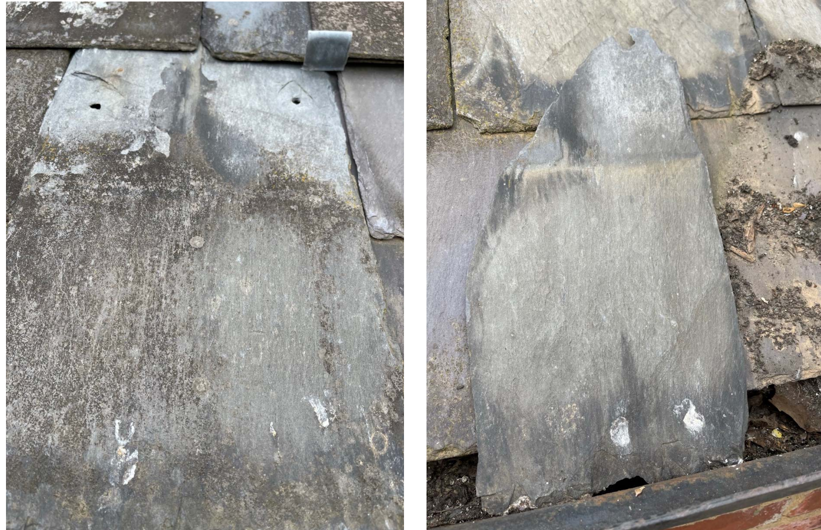
Slipped slates. Typical in numerous locaitons throughout the roof. Indicitatve of nail rot.
