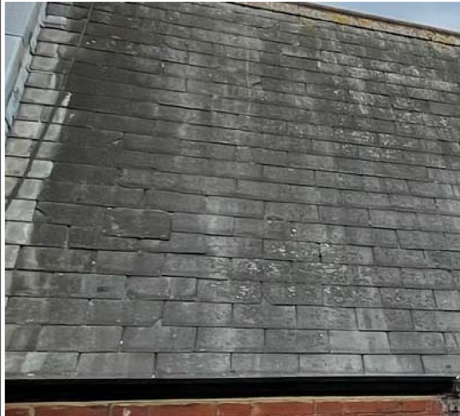
Slipped and broken slate.
