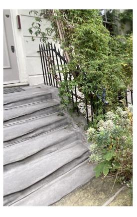
Existing steps covered in asphalt that has been poorly lain and has therefore melted, potentially causing trip hazard
