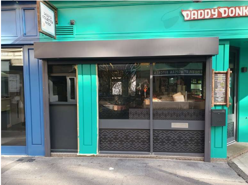
Image below of Leather Lane Shopfront with shutters in open position
