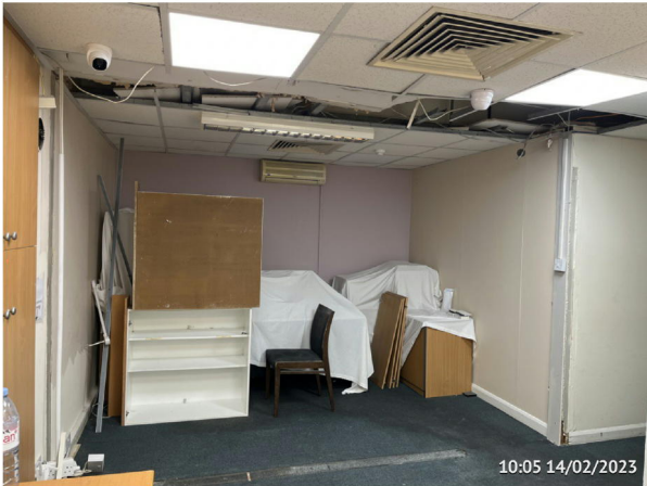
Item 4 Location Basement All largely demolished works ongoing
