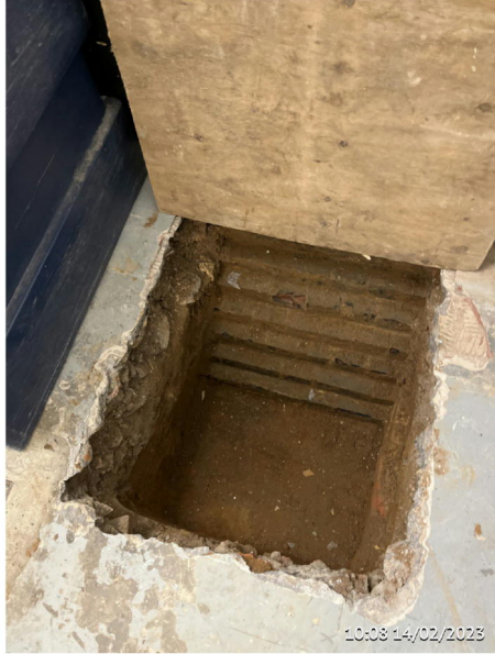
Item 5 Location Basement Foundation works ongoing
