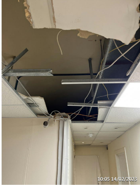
Item 3 Location Basement Demolitions ongoing
