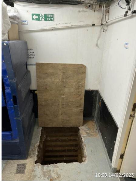
Item 7 Location Basement Foundations started.
