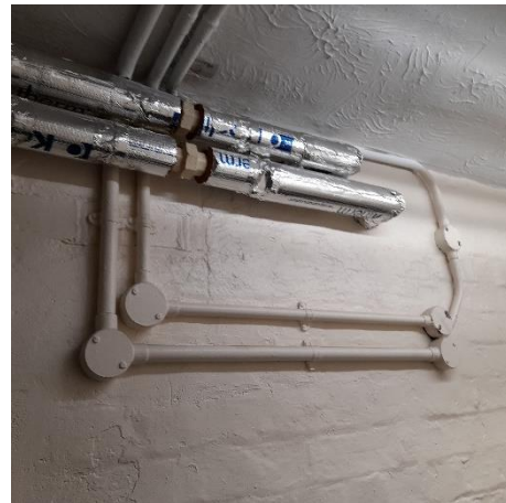
Photo 26 – Cable containment through wall into boiler room
