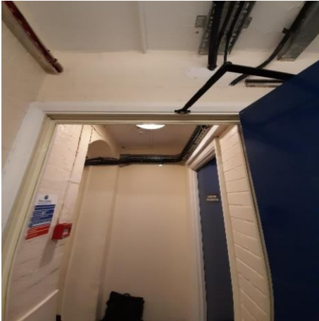
Photo 17 - Cable/ Cable Tray Penetrations Through Wall in Corridor
