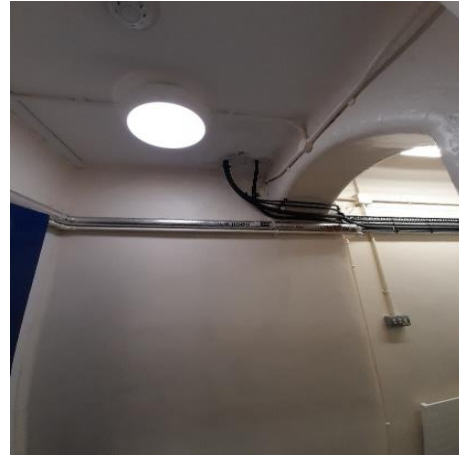
Photo 18 - Cable Penetrations Through Ceiling in Corridor
