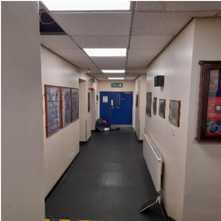
Photo 19 - Damaged/ Missing Ceiling Tiles to be Replaced (like for like)
