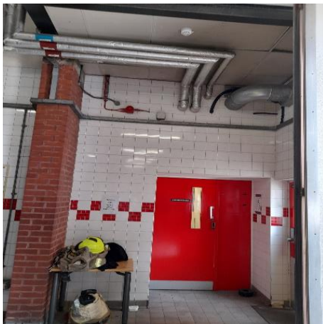
Photo 9 - Piped Services Penetrations and Ventilation Duct Through Wall in Appliance Bay
