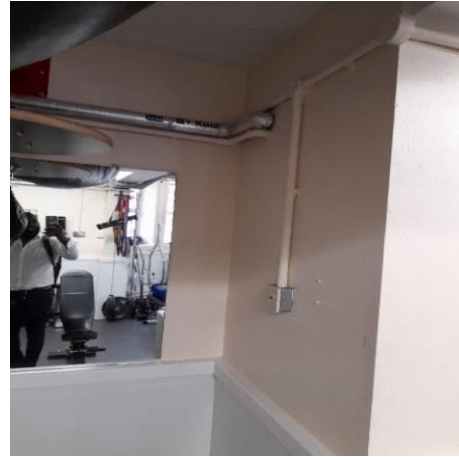
Photo 8 - Piped Services Penetrations Through Wall in Gymnasium
