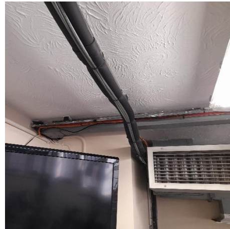
Photo 24 – Cable containment through wall at high level into gym from main switch room
