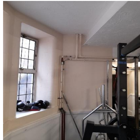
Photo 12 - Piped Services Penetrations to Above in Gymnasium
