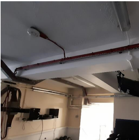
Photo 25 – Cable containment at high level in gym
