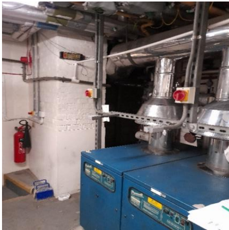
Photo 1 - Services Riser in Boiler room
