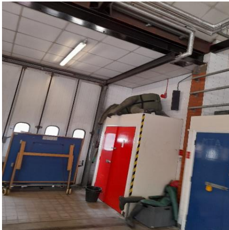
Photo 11 - ASHP Piped Services Penetrations Through Appliance Bay Internal Wall
