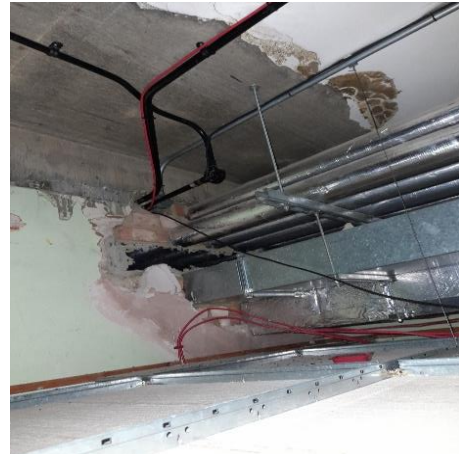
Photo 20 - Piped Services and Cable Penetrations Through Wall in Ceiling Void
