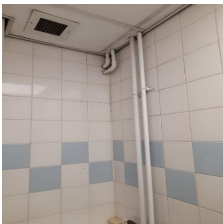
Photo 15 - Piped Services Penetrations from Above in WC
