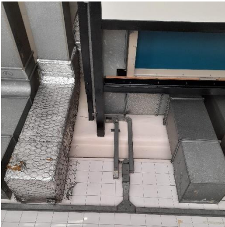
Photo 23 – Cable containment through wall at high level into appliance bay
