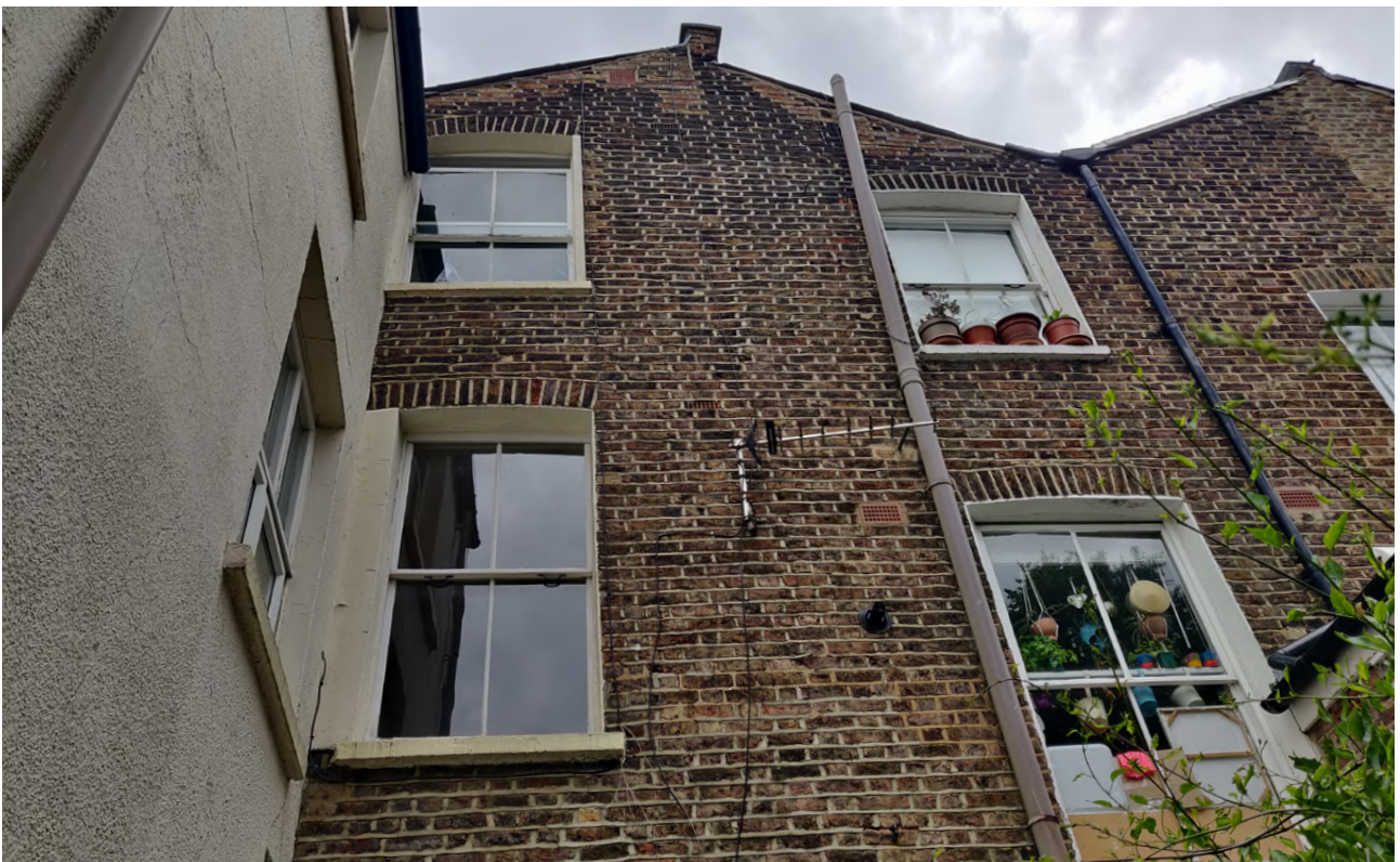
[Fig. 07] Rear (south-west) elevation with rendered outrigger seen to the left. Rear elevation windows to be replaced with new thermally efficient sliding timber sash windows in style and colour to match existing
