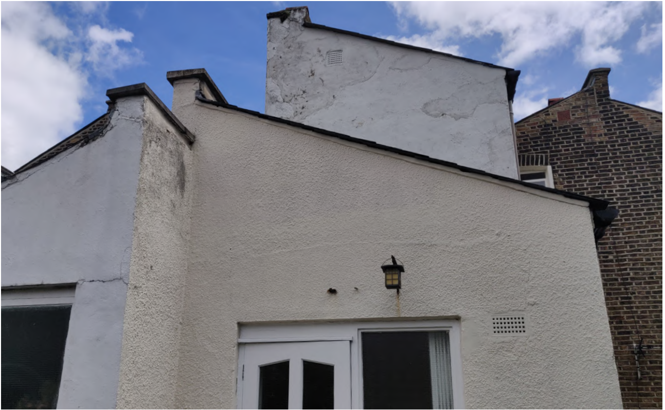
[Fig. 10] General refurbishment work needed to external elements such as render finish at rear. Patch render repairs to prevent water ingress as required with finish and colour to match existing
