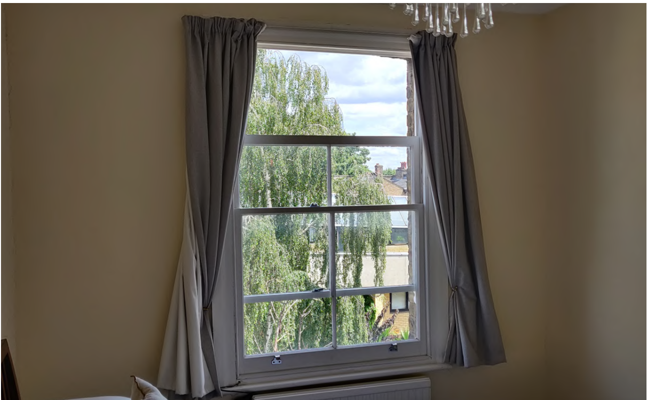
[Fig. 17] Existing Bedroom window replaced with new thermally efficient sliding timber sash window in style and colour to match existing
