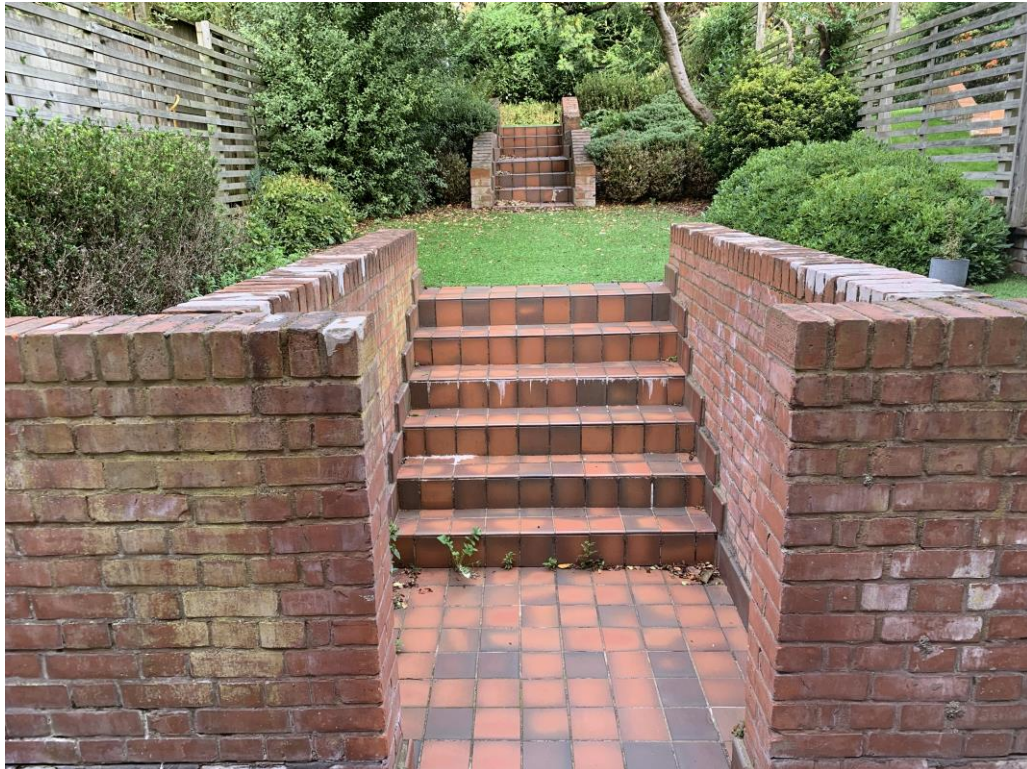
P4: current stepped arrangement into the garden
