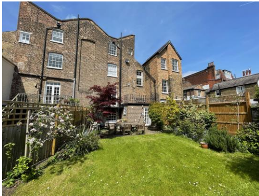
Figure 10: The rear façade of nos.44 and 45 Downshire Hill.
