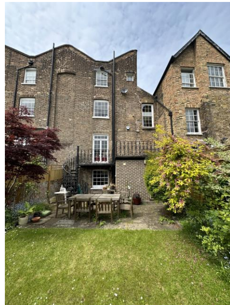
Figure 21: The current appearance of the rear façade with the 1980s extension adjacent to the modern cast iron balcony and spiral staircase.
