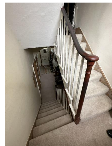
Figures 14-16: The ground floor hallway, ground floor fire surround and main staircase.
