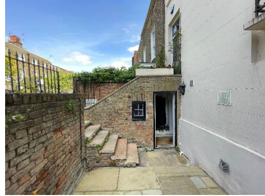
Figure 23: The existing rebuilt front lightwell area and steps.
