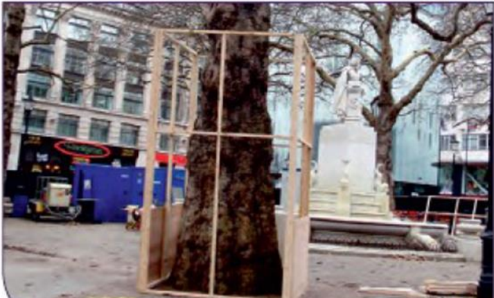
A wood frame around the trunk can be used to support a plywood surround.
