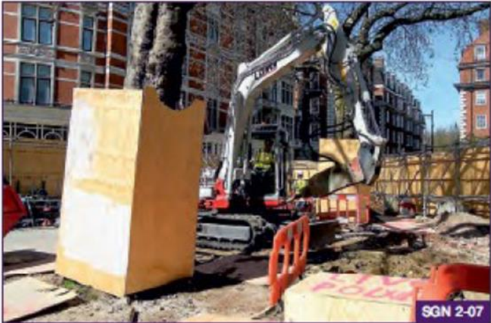
Boards attached to a supporting framework surrounding the trunk reduces the risk of accidental impact.
