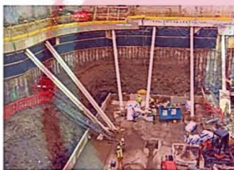
Typical temporary propping layout with bespoke construction sequencing
