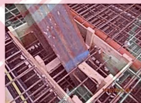
Temporary propping may result in bespoke waterproofing details around the propping elements.
