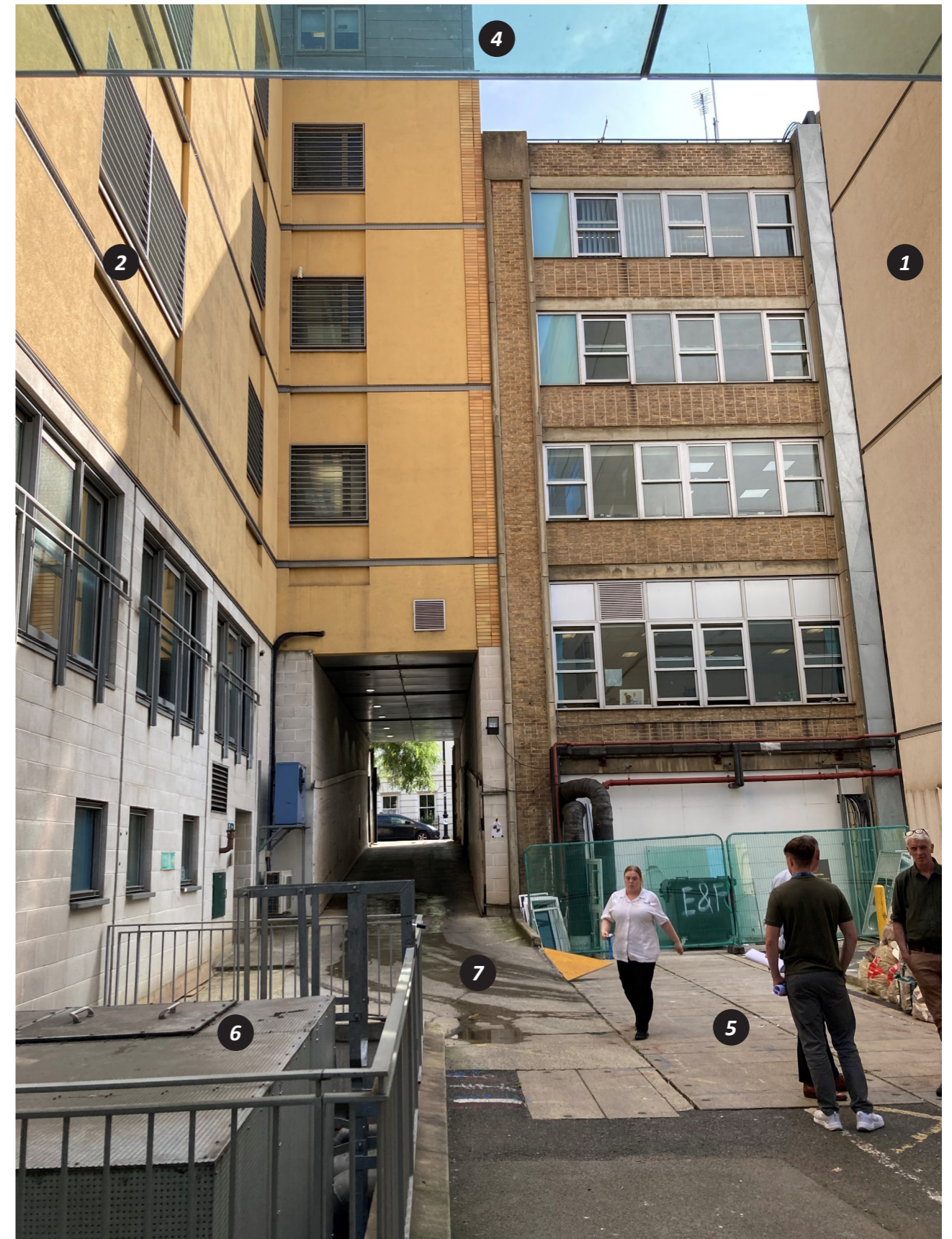
Photograph taken from within the services yard facing south, 2023
