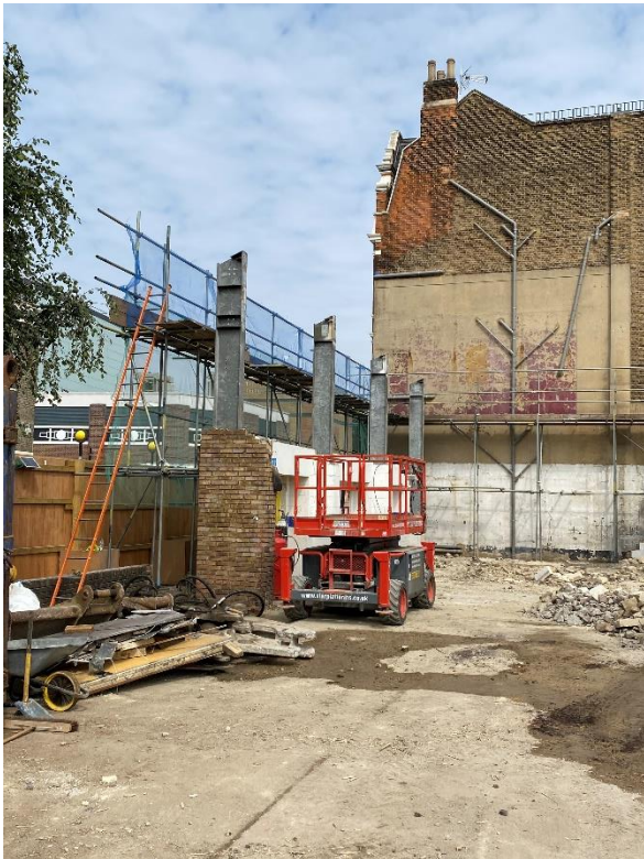
Remainder of RCS Facade
