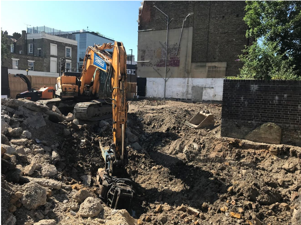
Obstruction Removal and Boundary wall Footing Projection
